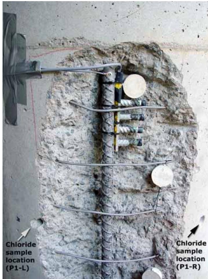
**Figure 8. Sacrificial Anode Monitoring Device Placement Before Shotcrete Repair**
