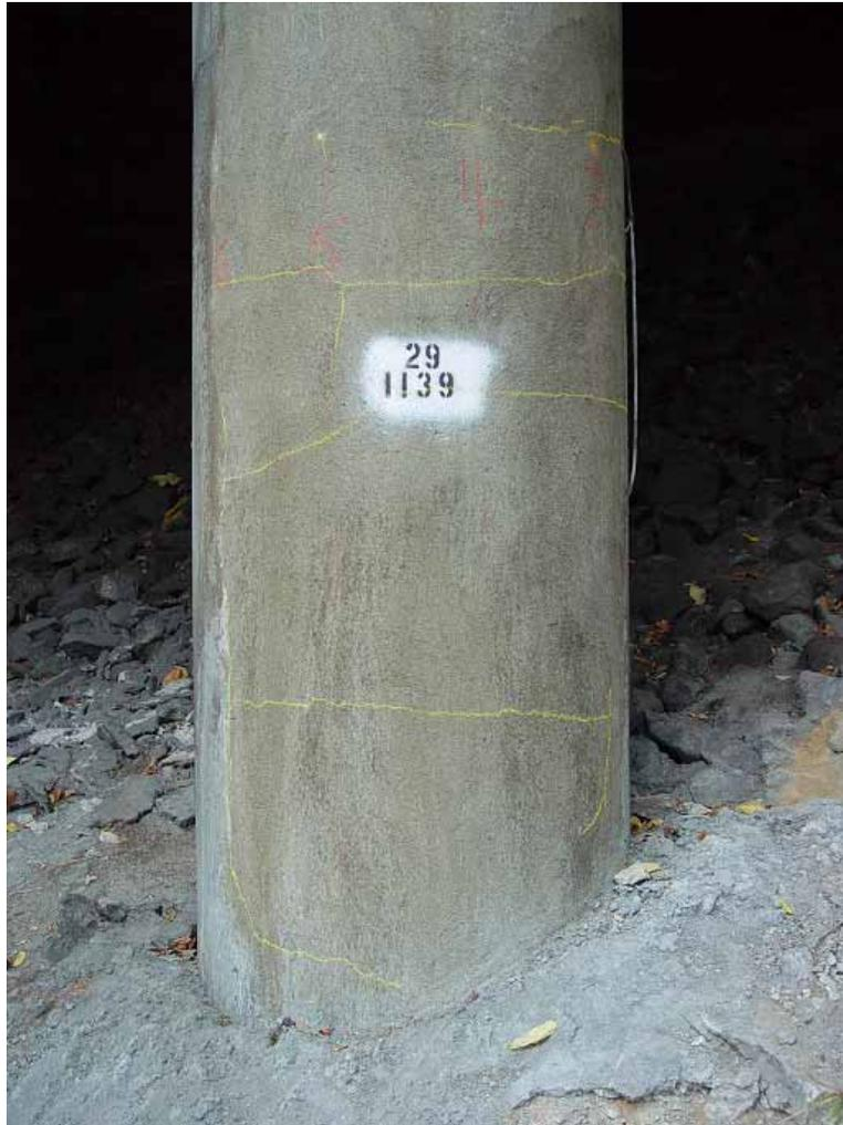
**Figure 10. Pattern of Small-width Cracks in a Shotcrete Column Repair**
