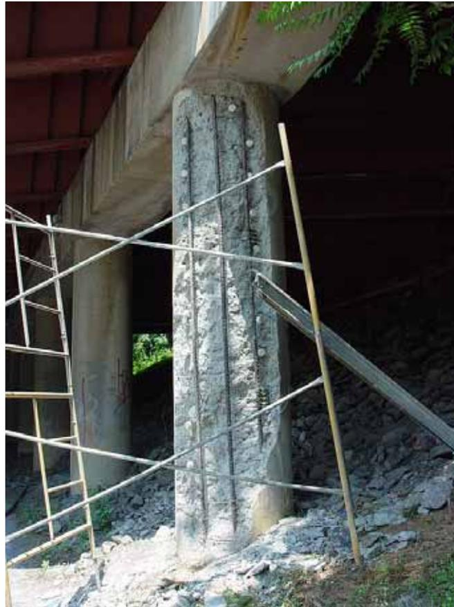
**Figure 3. Placement of Anodes in Shotcrete Repair Areas**
